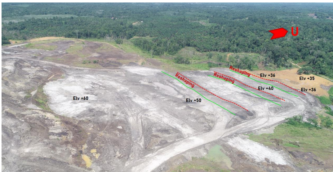
Gambar 15. Proses Lift Up RL+40 – RL+60
